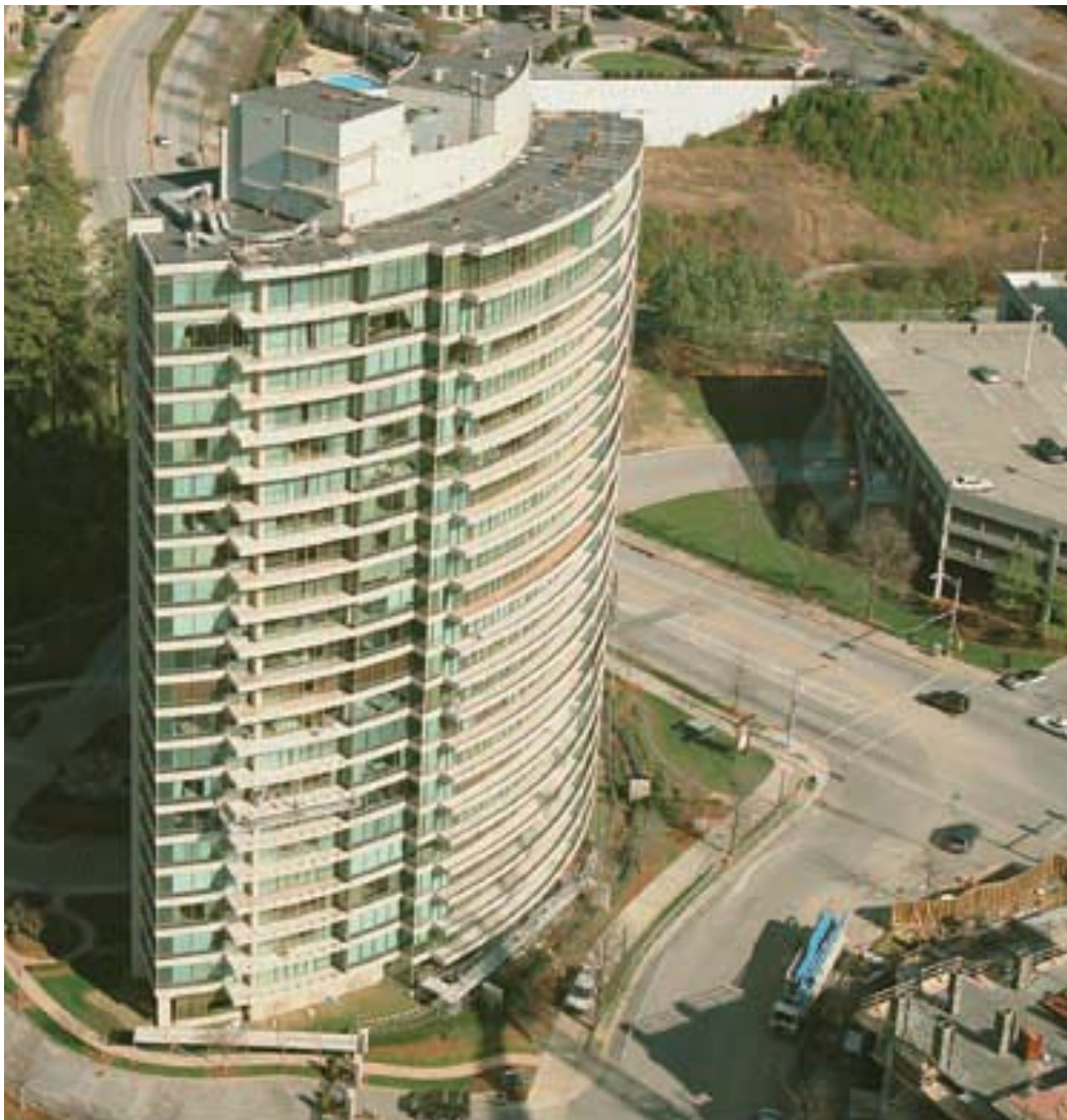
The Park Regency condominiums in Buckhead are one of Morley's show case projects for concrete restoration and waterproofing.
